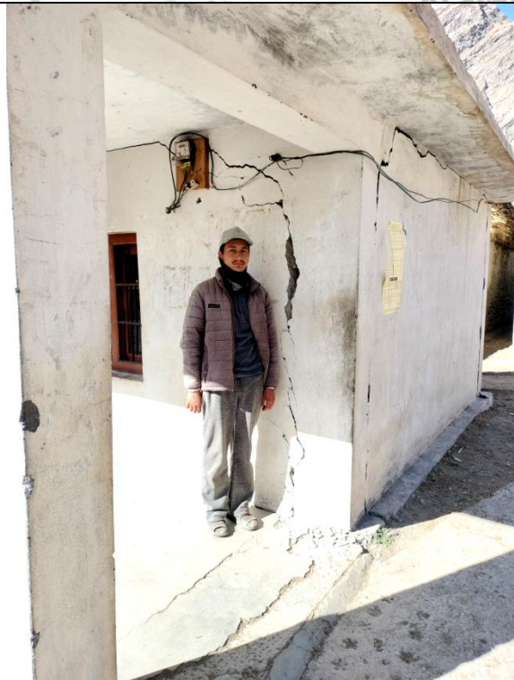
Fig. 20: Ground cracks continuing into the walls of a community centre. Note that the trend of cracks on the wall and ground is same.
