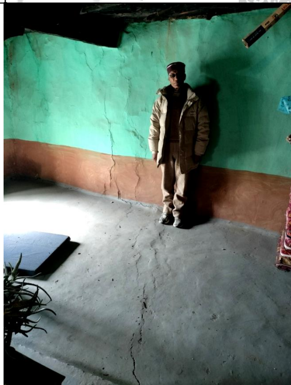
Fig. 16: Cracks on the floor of a mud house can be seen continuing towards the wall.
