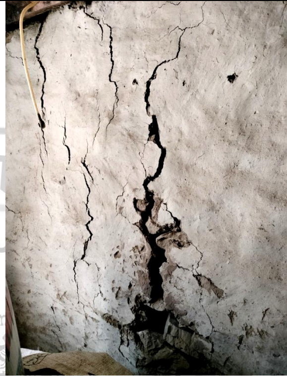
Fig. 19: Highly damaged and bulged wall of an old mud house (~80 years old).
