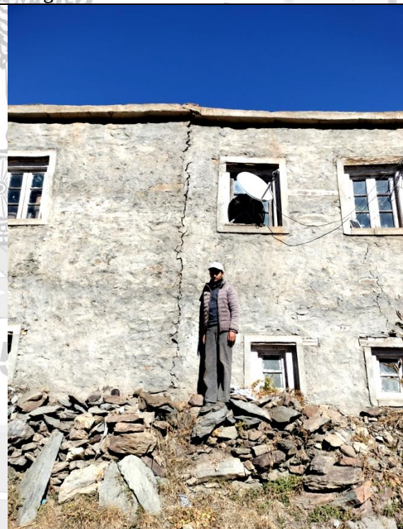
Fig. 17: Subsidence near the house has led to the formation of irregular vertical cracks.
