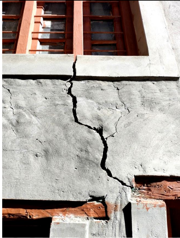
Fig. 18: Step cracks with 2.6 cm opening seen in a mud house.
