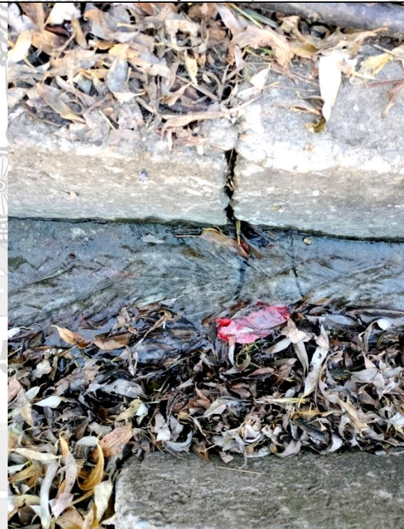
Fig. 21: Vertical cracks observed in a man-made channel with flowing water near a house leading to possible seepage of water to the ground.
