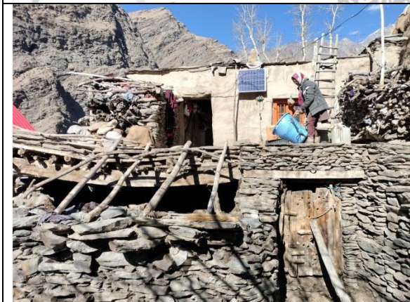
Fig. 12: 80 year old highly damaged mud house built on rock piles with no proper foundation.
