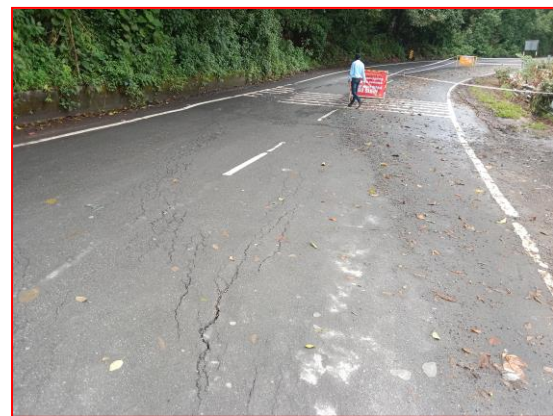
Fig 9: Subsidence with curvilinear cracks of NH181 road near Nadu Gudalur
