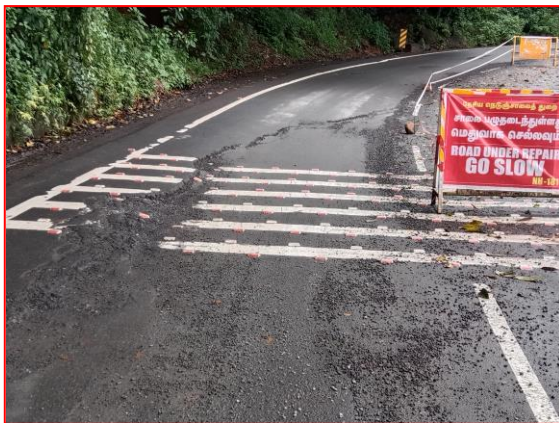
Fig.8: Subsidence of NH 181 road near Nadu Gudalur
