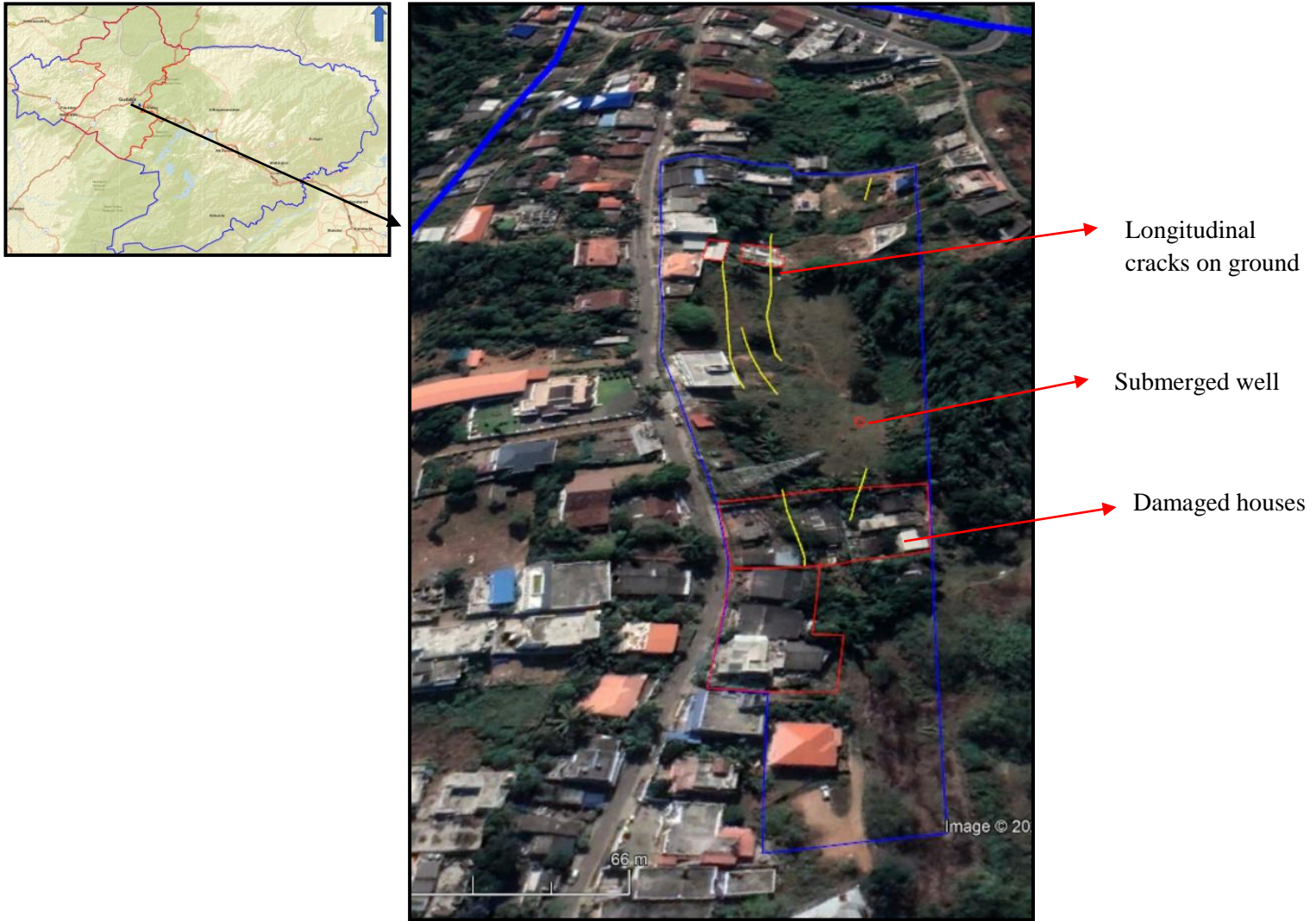
Fig: 2. Plain view of study area showing landslide location area showing cracks
